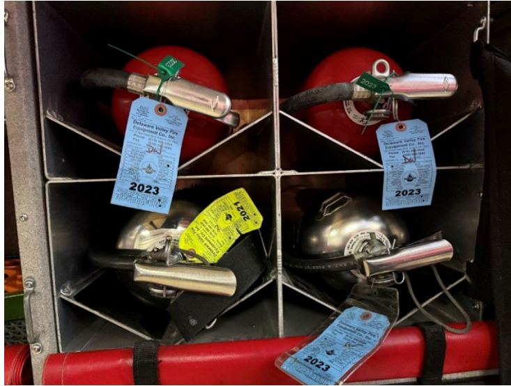
Fire Extinguishers are out of date and need to be recertified.
