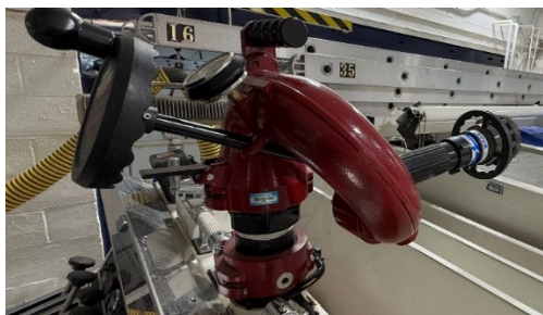
Replace the combination nozzle with a set of stacked tips with a smoothbore and a stream shaper to achieve reach and penetration of the stream.
