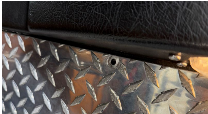
Areas were noted to be missing screws. These areas need to be identified and repaired.
