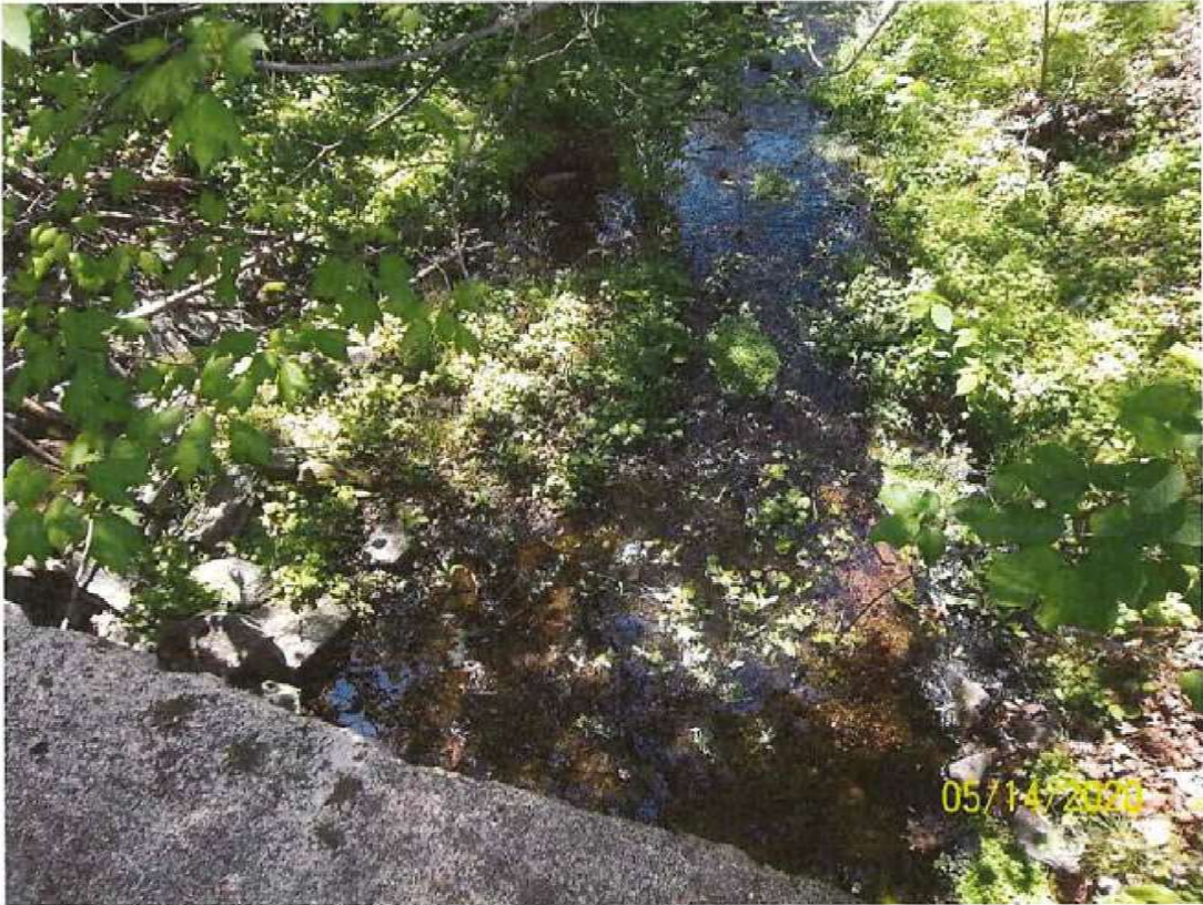
Figure 22. Other side of culvert under Putters Lane.
