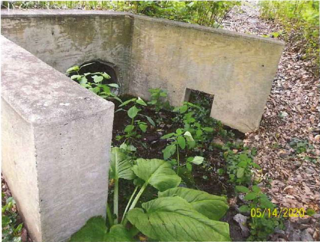
Figure 10. Culvert under the driveway of 2 Brookside Road.
