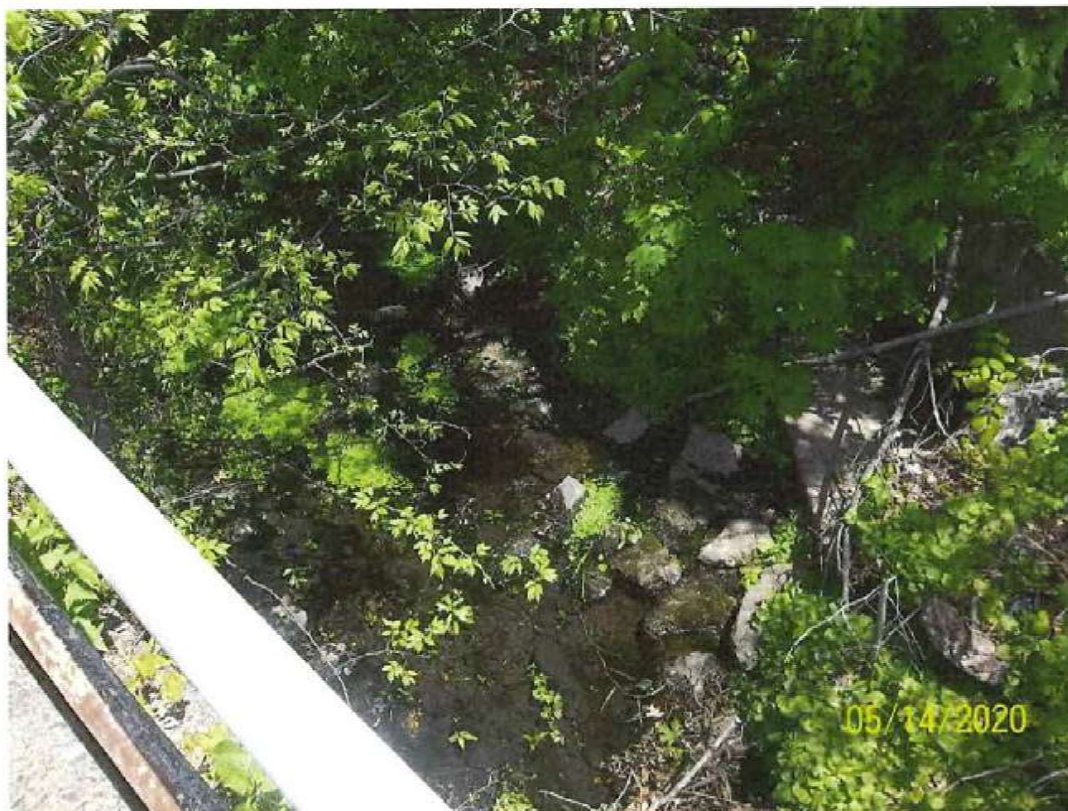
Figure 23. Tributary crossing under Providence Road.
