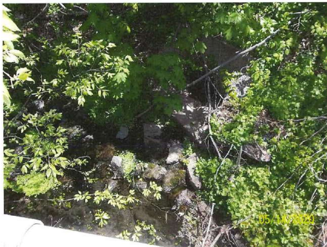
Figure 24. Tributary crossing under Providence Road.
