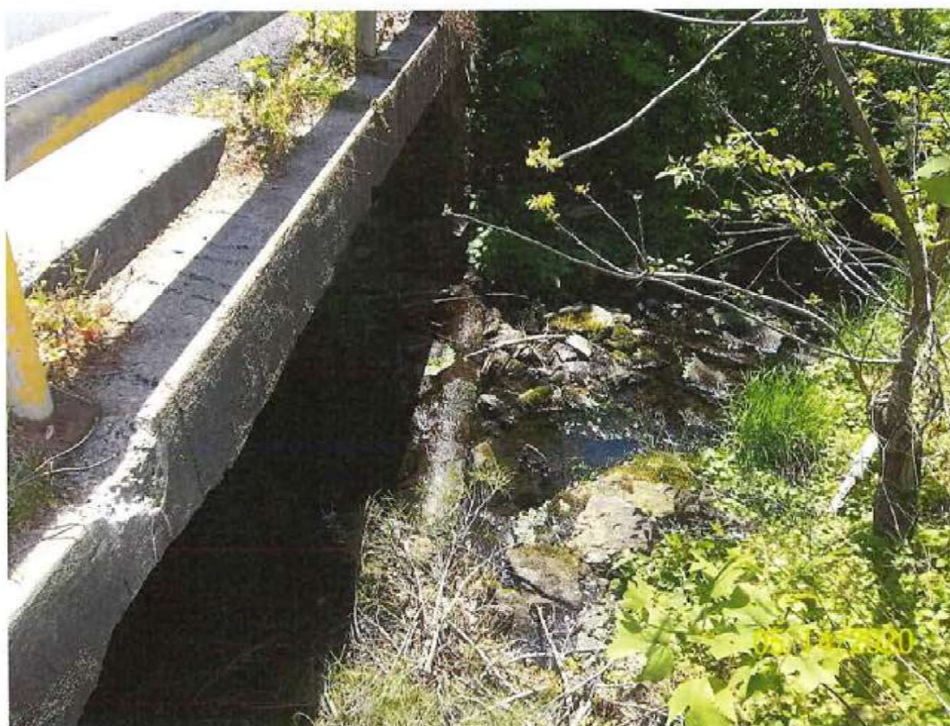
Figure 26. Other side of culvert under Providence Road.
