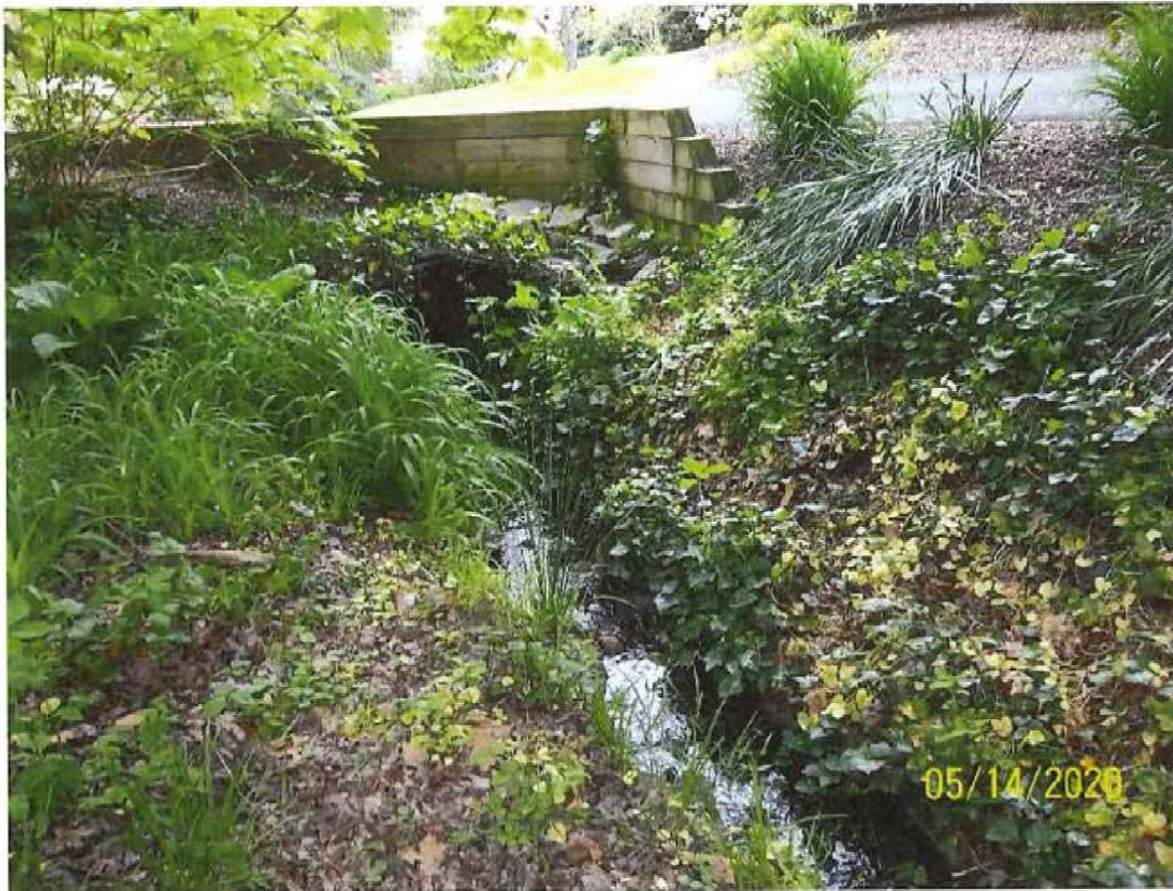
Figure 15. Continuation of Vernon Run Tributary past the driveway of 212 Fox Lane.
