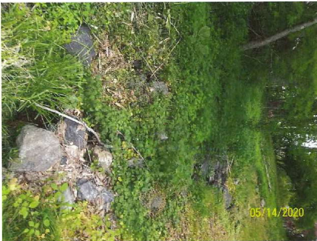
Figure 22. Flowing water is buried by rocks and seems to go underground. Third Branch ends about 60 ft past 211 Fox Lane.
