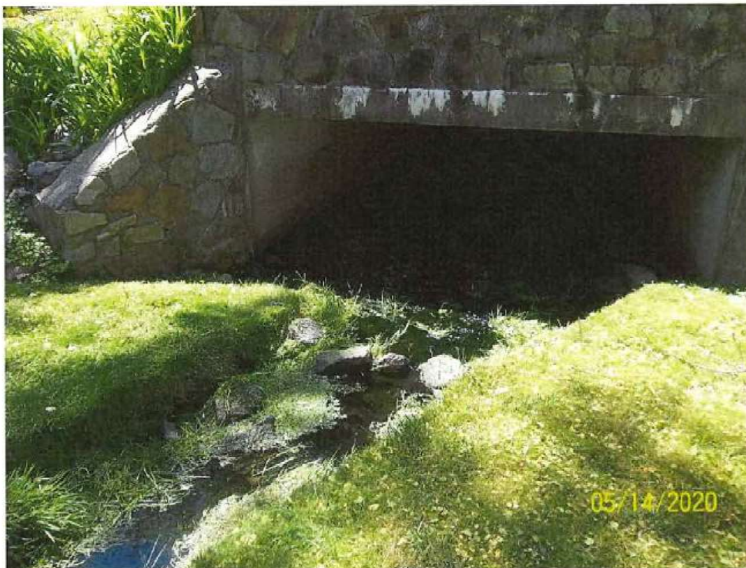
Figure 19. Culvert under Putters Lane.
