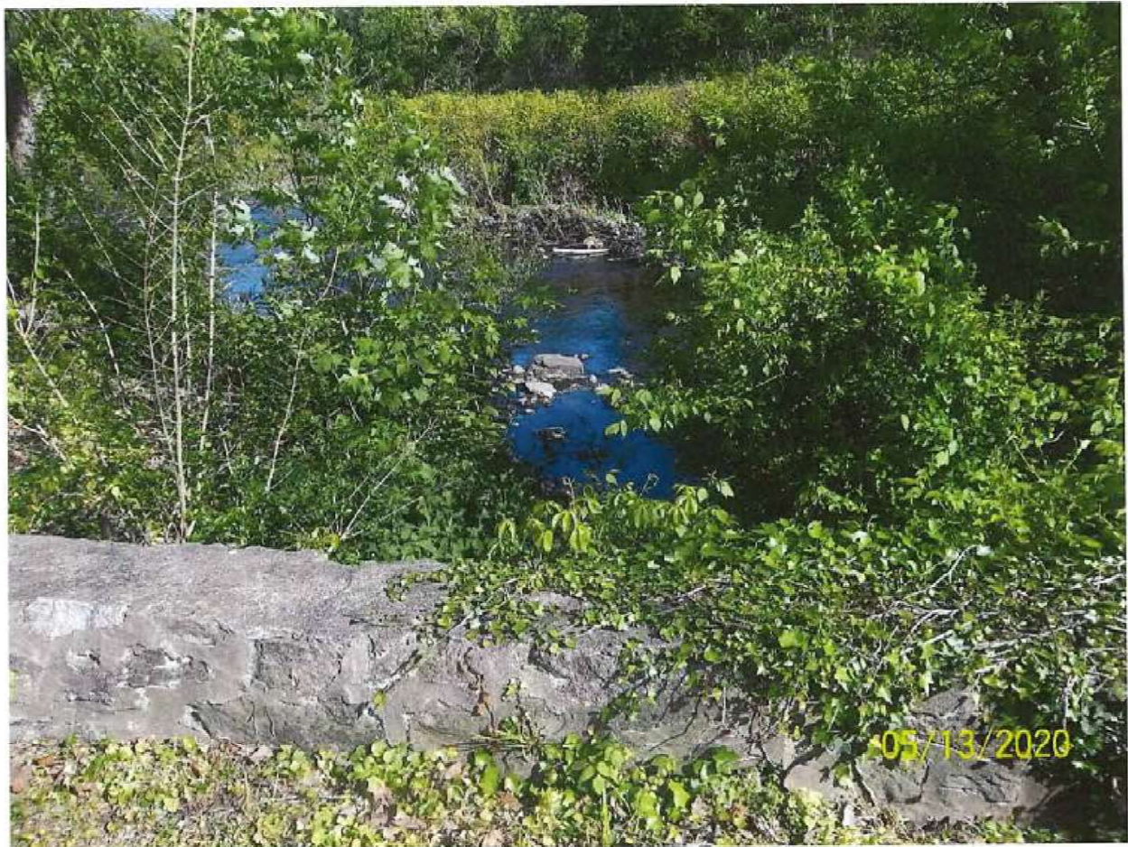
Figure 29. Top of culvert discharging to Ridley Creek on the other side.
