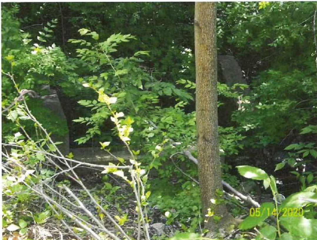
Figure 10. Side image of culvert.
