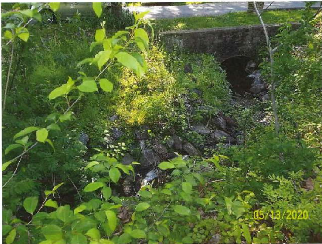
Figure 20. Closer image of culvert under Bullens Lane.
