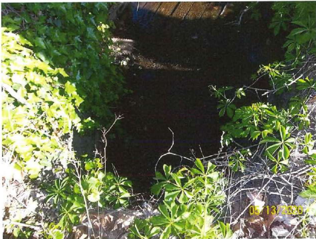
Figure 22. Other end of culvert where tributary resurfaces above ground.
