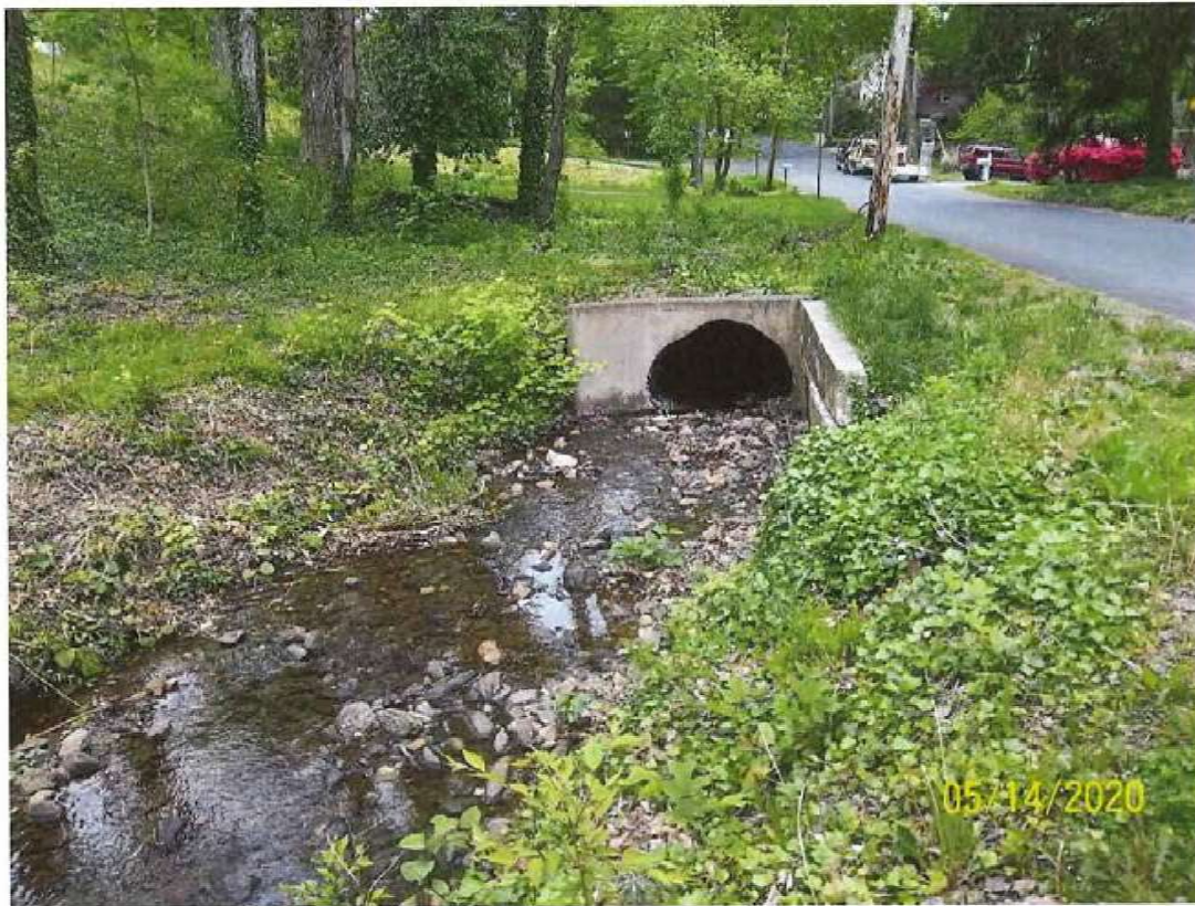
Figure 23. Pine Ridge Run crossing under Pine Ridge Road.
