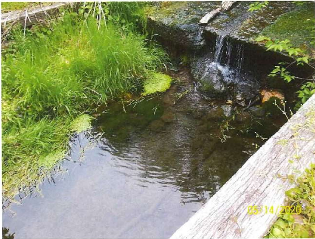
Figure 13. Flowing water in front of the culvert.
