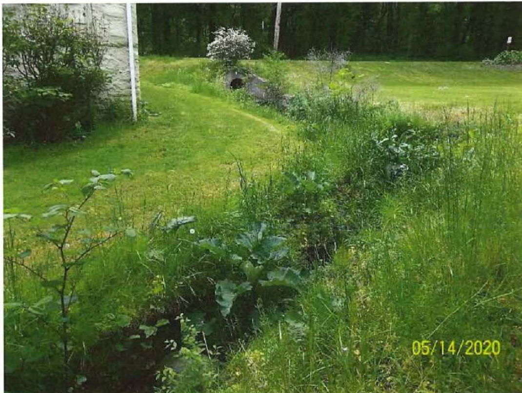
Figure 14. Tributary flowing down from the culvert.
