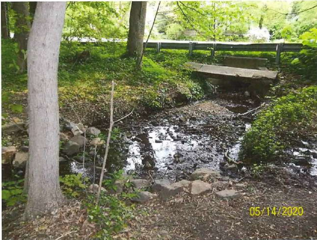
Figure 9. Tributary crosses underneath Turner Road.
