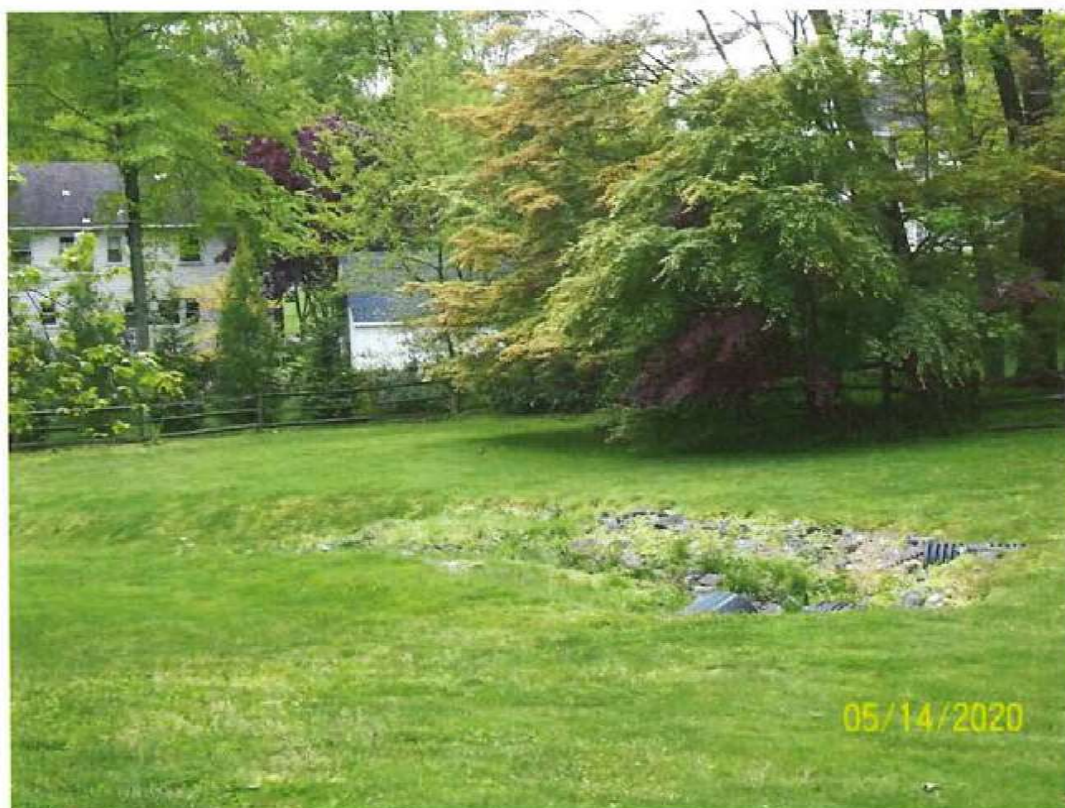
Figure 2. Multiple pipes discharge in location to the left of the street in Figure 1.
