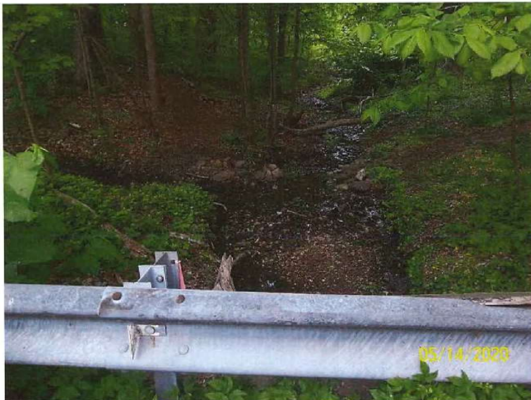
Figure 10. Tributary crosses underneath Turner Road.
