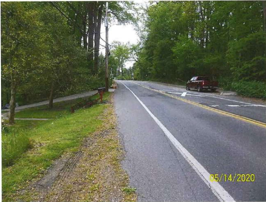
Figure 11. Turner Road where the Tributary crosses underneath.
